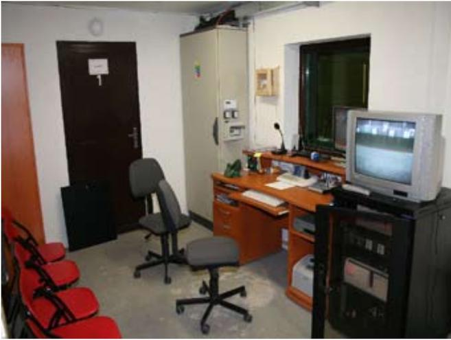
Control room with bullet-proof window, audio, video, rack with controlling electronics. To left main switchboard, control device for air-conditioning.
