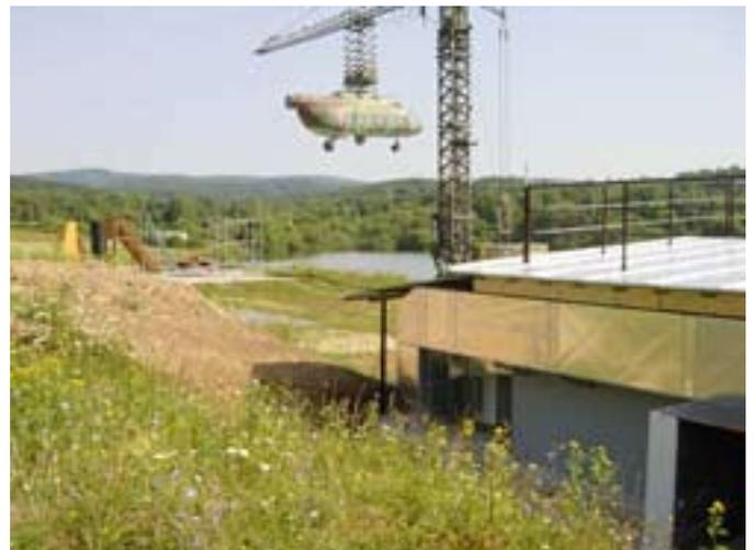
Door and window access points into the tactical part of the building. Flat roof with ladders and solid railing. Side windows and doors adjusted for shooting inside of the shooting range.
