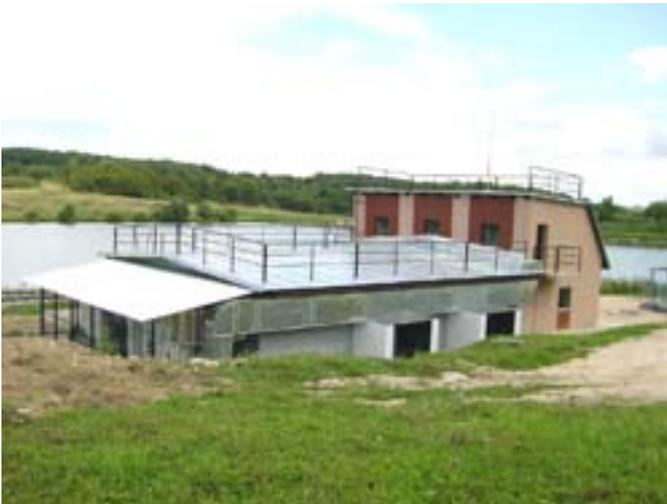
Side low windows for shooting inside, above these is air-condition pipe, below the air-condition module and ventilation for the shooting range
