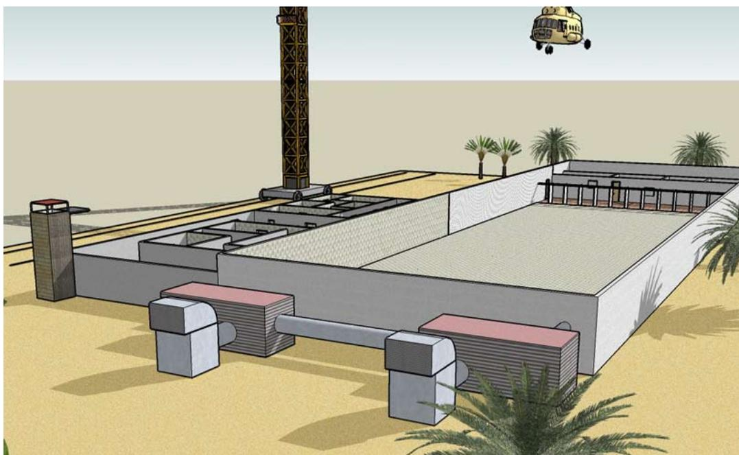
Powered ventilation and air conditioning equipment can also be seen in the picture. At full power it must ensure exchange of all the air inside the shooting range 30 times in one hour. The ventilation system protects the user against the danger of air pollution from shooting.
