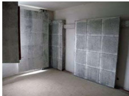
The walls of the rooms are protected by ballistic only where necessary. At some places the ballistic protection of sliding along the wall
