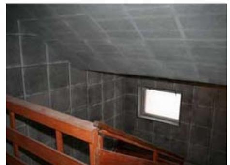
Hallway are fitted with the same ballistic protection as the rooms
