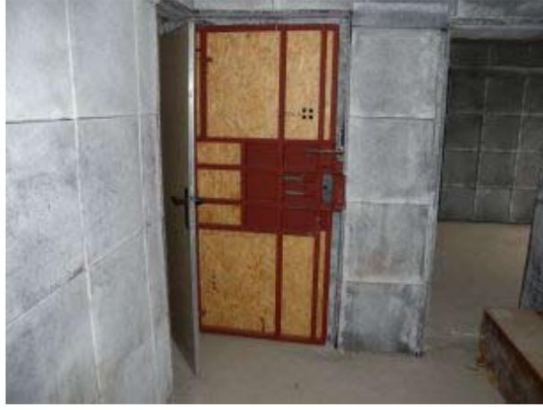
Some rooms are equipped repeated breachable doors, which are designed to train the technique of forced entry. Allow forced entry in several ways.
